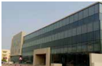
Commercial Building C-Ring
